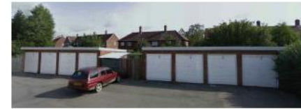
EXISTING SITE PHOTO
