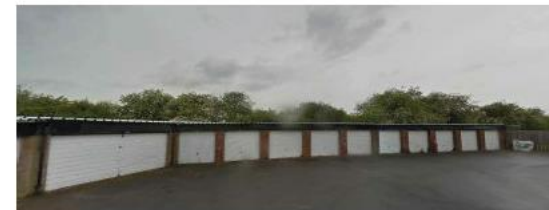
EXISTING SITE PHOTO
